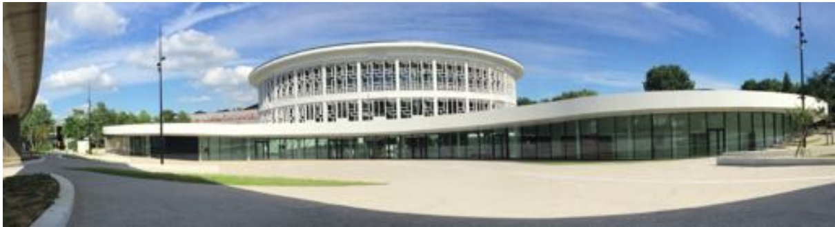
The new Lilliad buildings (Lille University Learning Center) on the Campus 'Cité Scientifique' at Villeneuve d'Ascq
